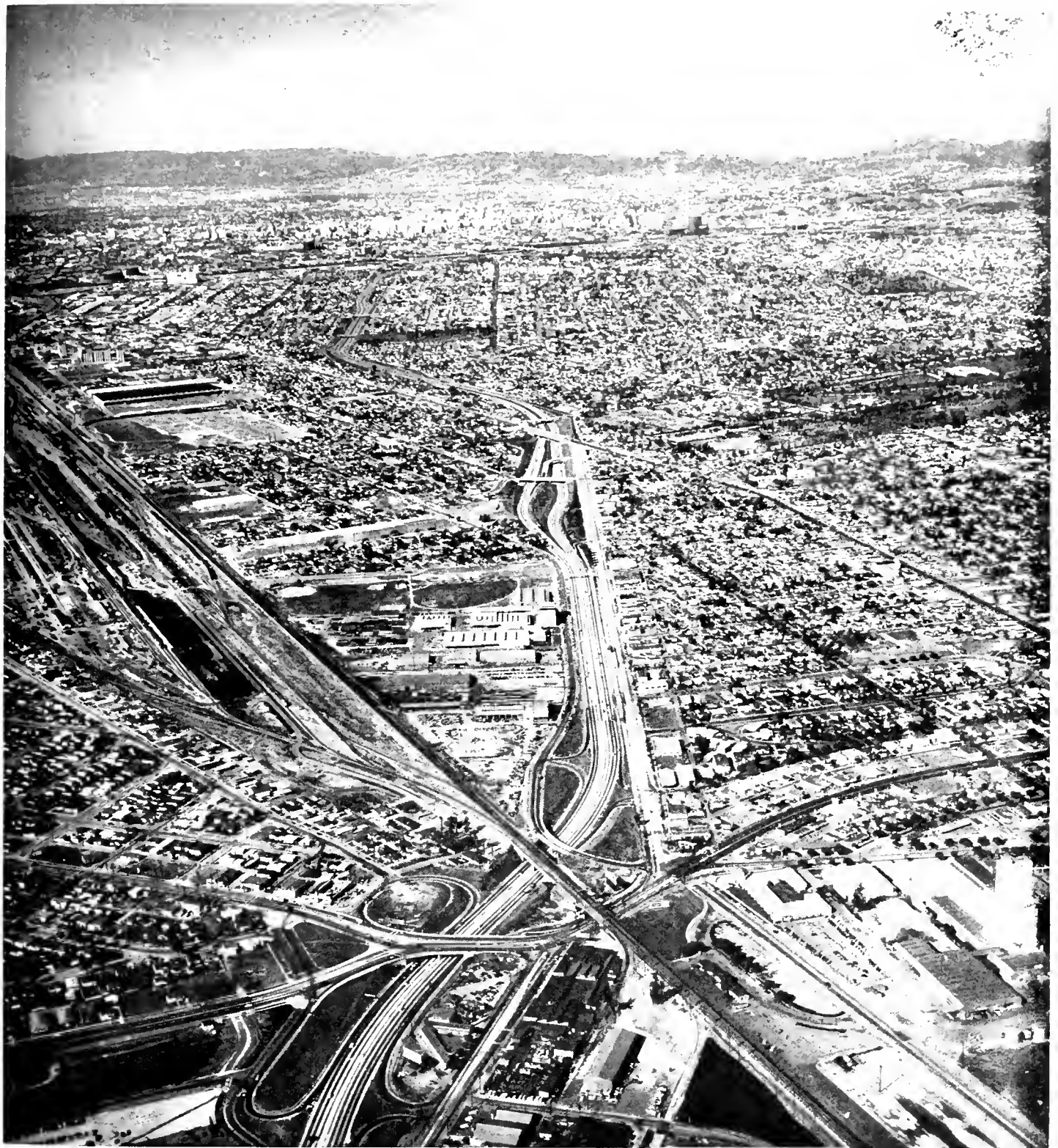
Looking northwesterly along completed Santa Ana Freeway, showing in foreground mixmaster interchange, with Atlantic Boulevard and Union Pacific Railroad being carried over the freeway
